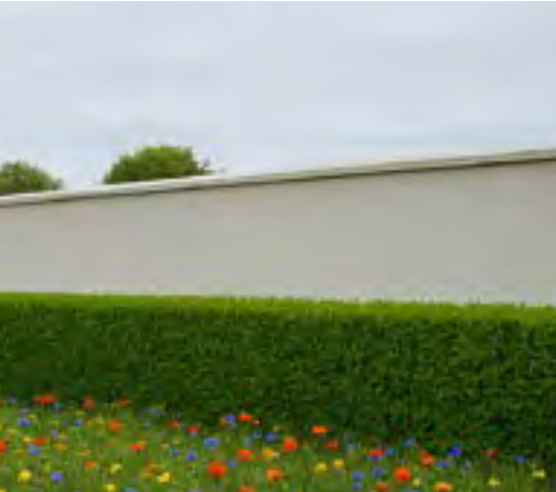
2.6M HIGH MASONRY BOUNDARY WITH CEMENT RENDER FINISH ON DEVELOPMENT SIDE AND DRY DASH FINISH ON ESB SIDE WITH CONCRETE COPING INCORPORATING ANTI CLIMB MEASURES 1.8M HEDGE TO BE INCORPORATED FOR SCREENING PURPOSE
